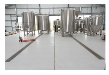
In July 2022, ACO KlassikDrain and ACO stainless channels, tailored to suit the specific needs of this craft brewery were installed enhancing safety, hygiene and efficiency at the same time. The installations serve distinct purposes within the facility.
